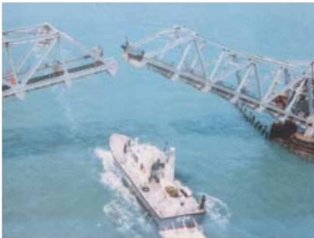
Coast Guard interceptor boat crossing the Pamban Viaduct
