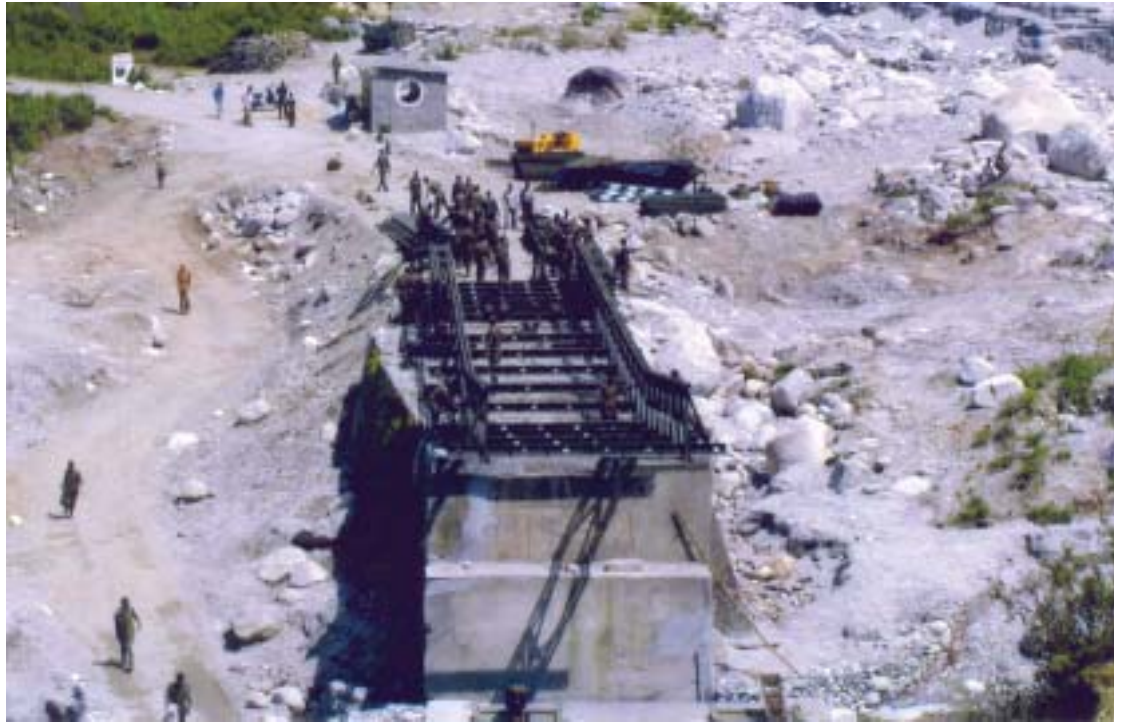
Army Jawans re-construct a bridge washed away during floods at Baijnath
